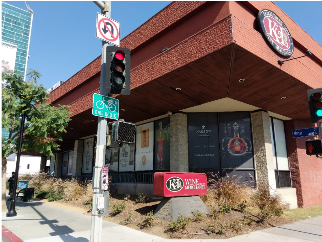
View of 1400 Vine Street structure to the northeast. 1400 Vine Street, Hollywood, California 90028
