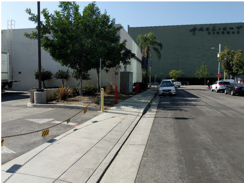
View of rear portion of 1440 Vine Street structure. 1440 Vine Street, Hollywood, California 90028
