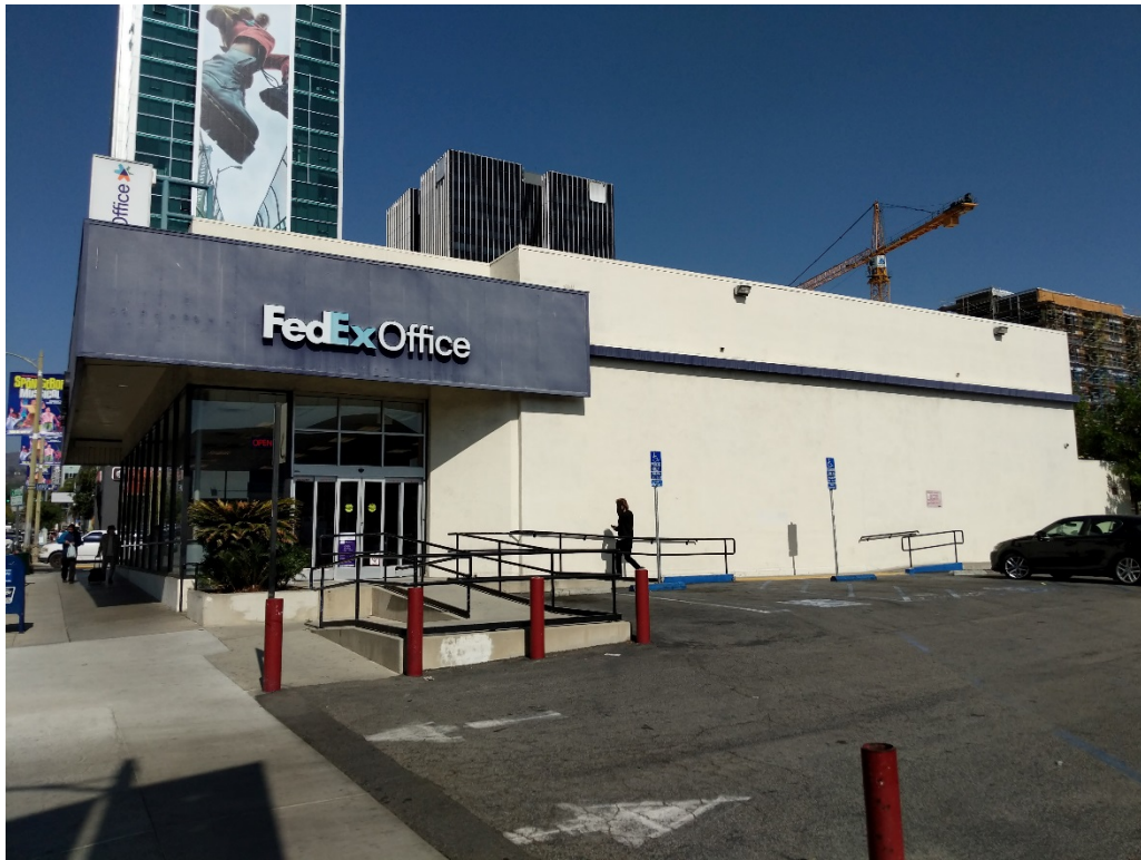
View of 1440 Vine Street structure to the northeast. 1440 Vine Street, Hollywood, California 90028
